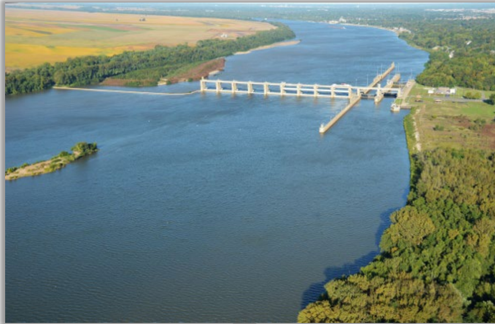
Image 27: Newburgh Locks and Dam
