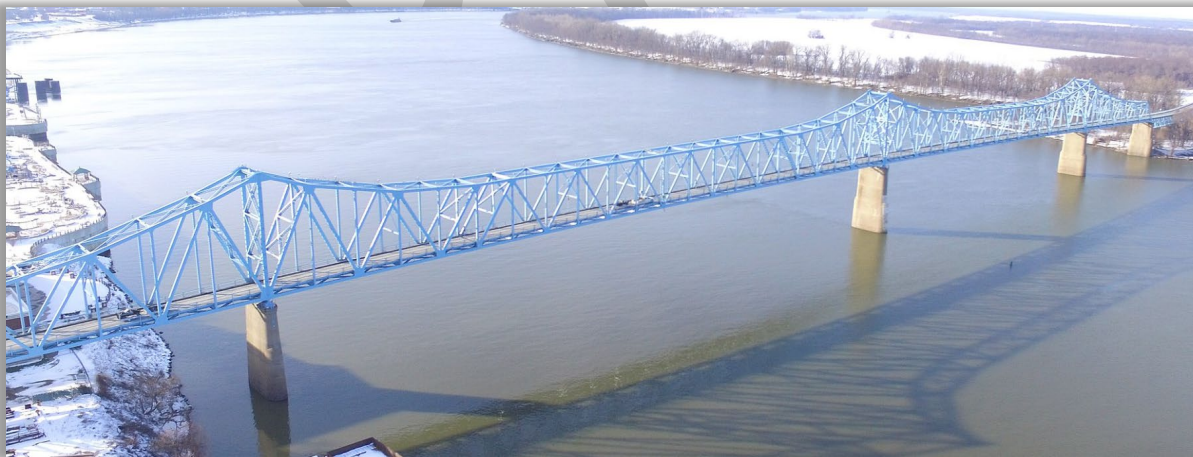
Glover Cary Bridge, Kentucky SR 2262, and Indiana SR 161
