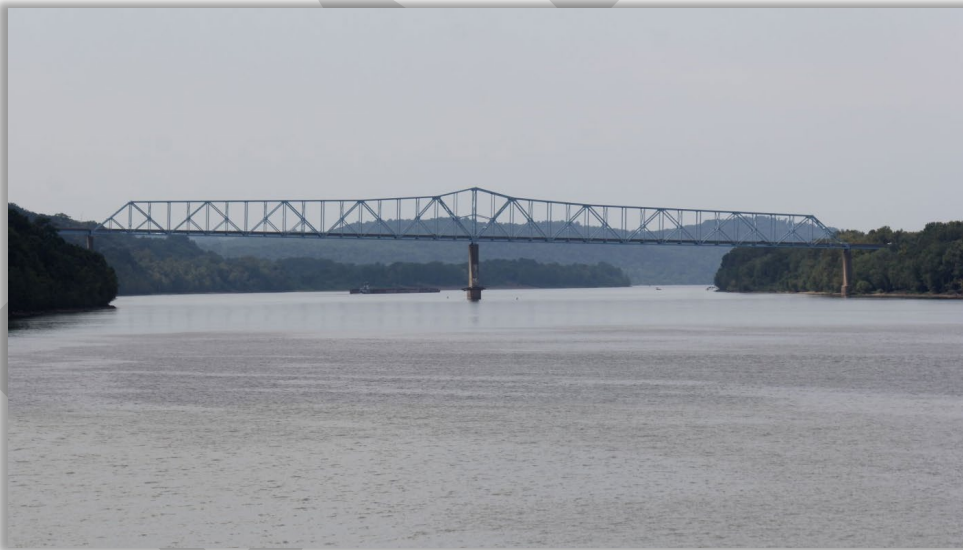
Image 18: Matthew E. Welsh Memorial Bridge, Brandenburg, Kentucky
