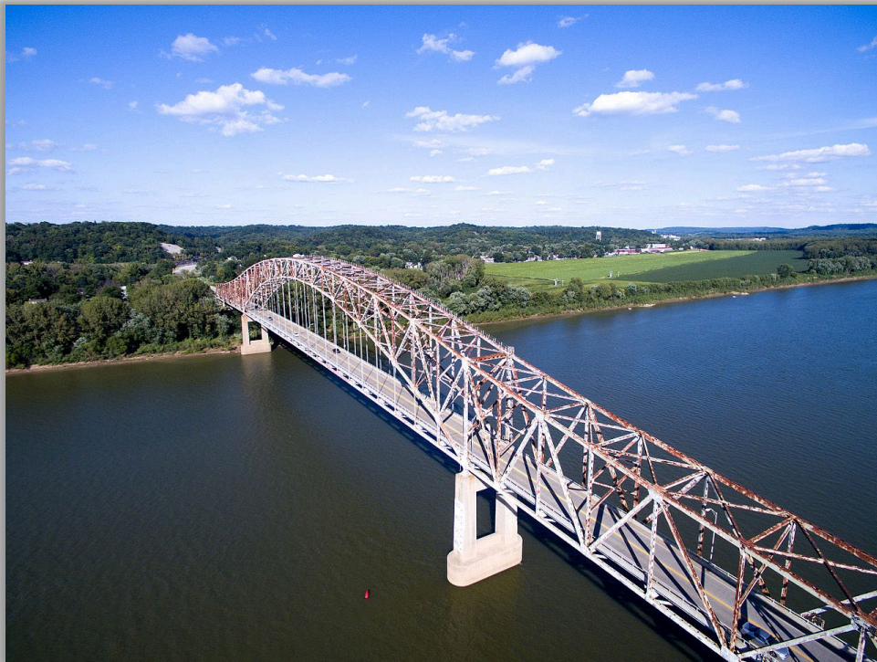
Image 19: Lincoln Trail Bridge, Cannelton, Kentucky
