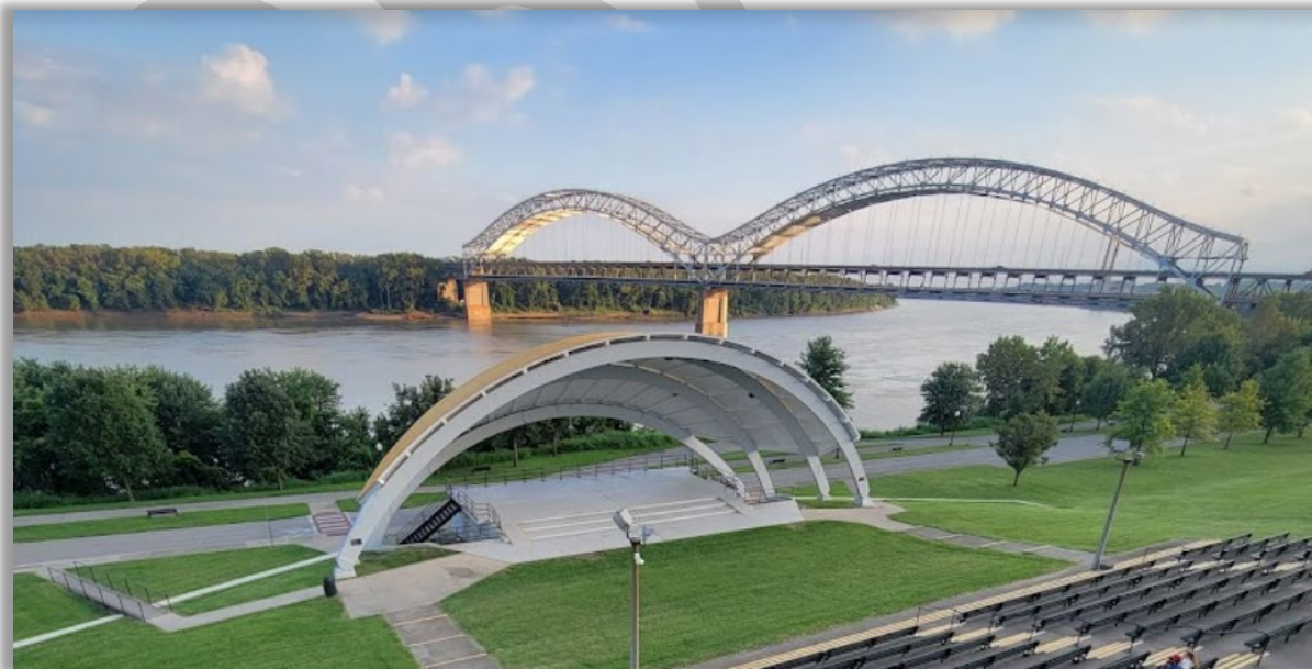
Sherman Minton Bridge, I-64, and US Hwy 50
