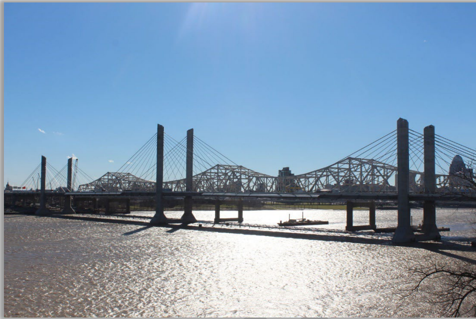
Image 11: Abraham Lincoln Bridge, Louisville, Kentucky
