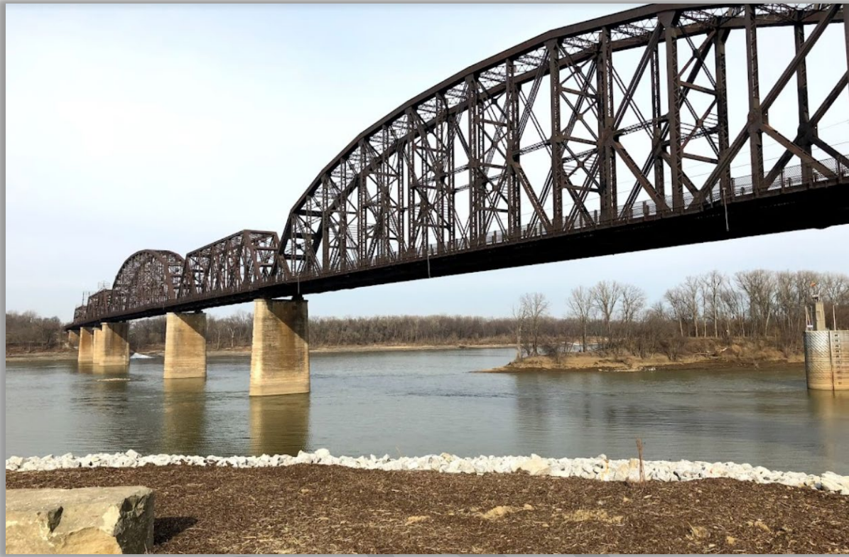
Kentucky and Indiana Terminal Bridge, Norfolk Southern track
