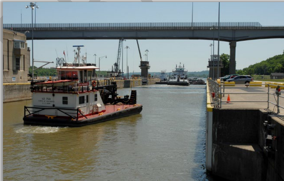
Image 24: Markland Locks and Dam
