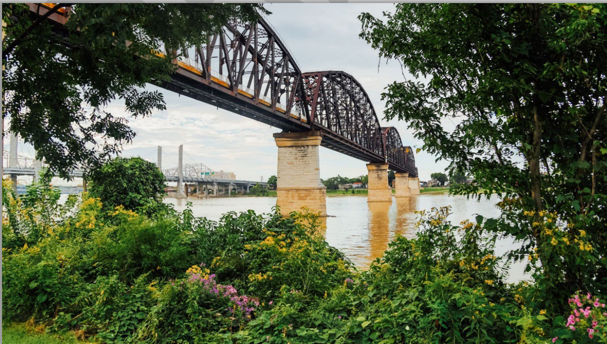
Big Four Pedestrian Bridge
